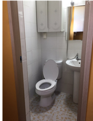
Bath room inside a room
